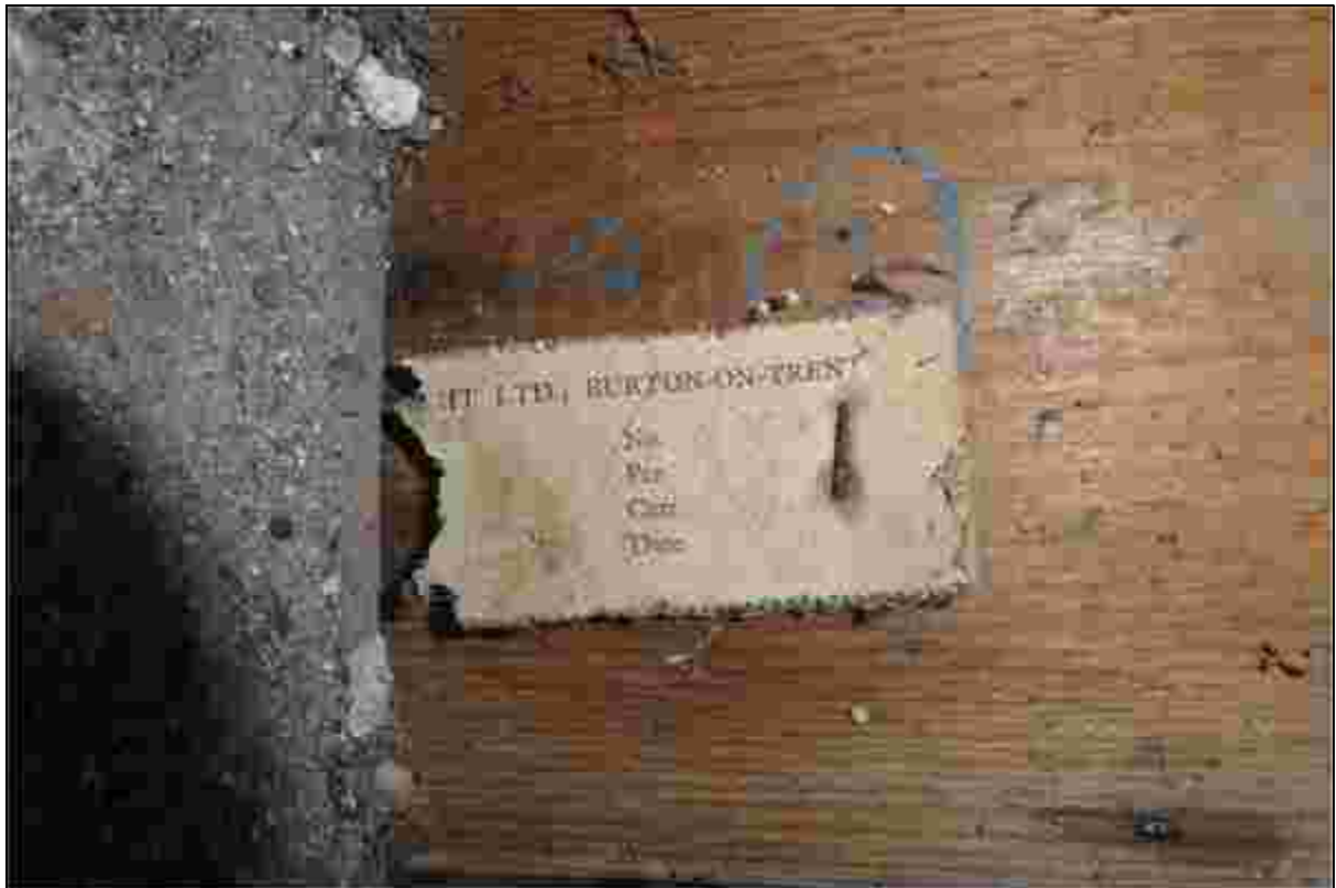
Plate 83: Paper label on the frame of the sash window in the western dormer
