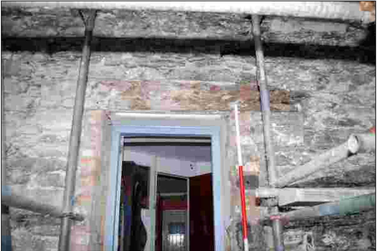
Plate 67: details of the wooden lintel over the front door.
