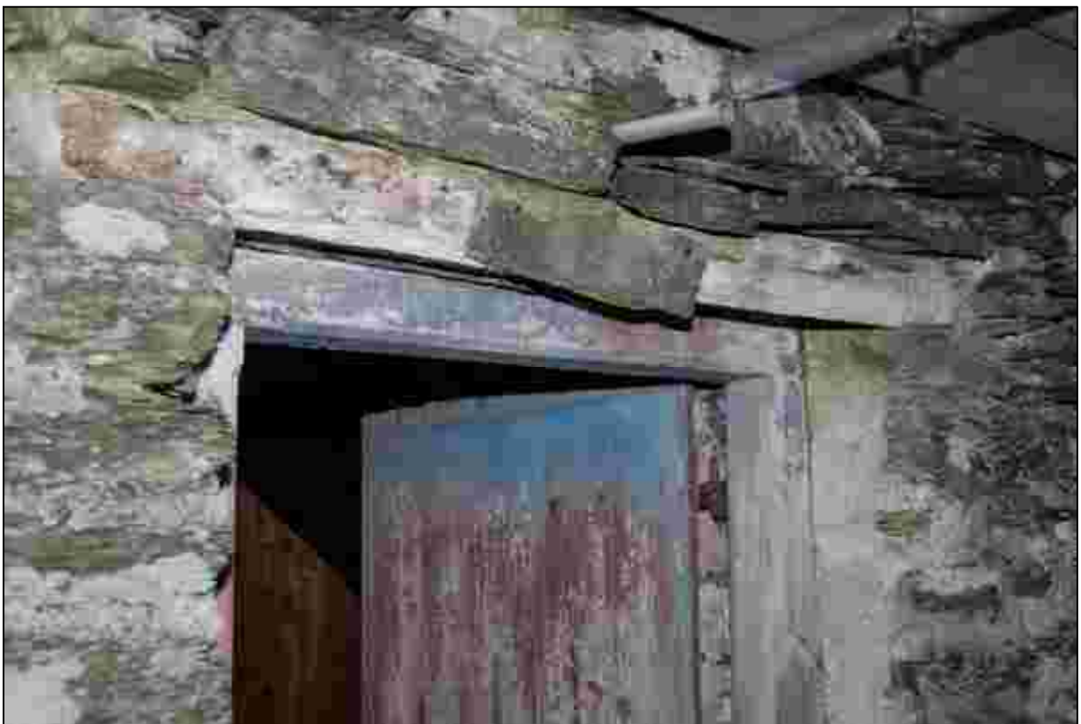
Plate 16: Lintel over the door in the eastern gable
