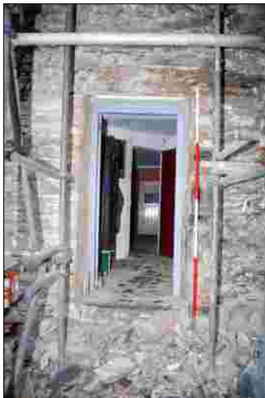
Plate 66: The front door after the removal of the render
