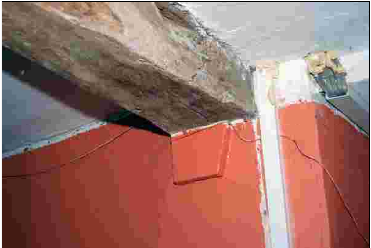
Plate 25: Chamfer and stop on the beam in the parlour
