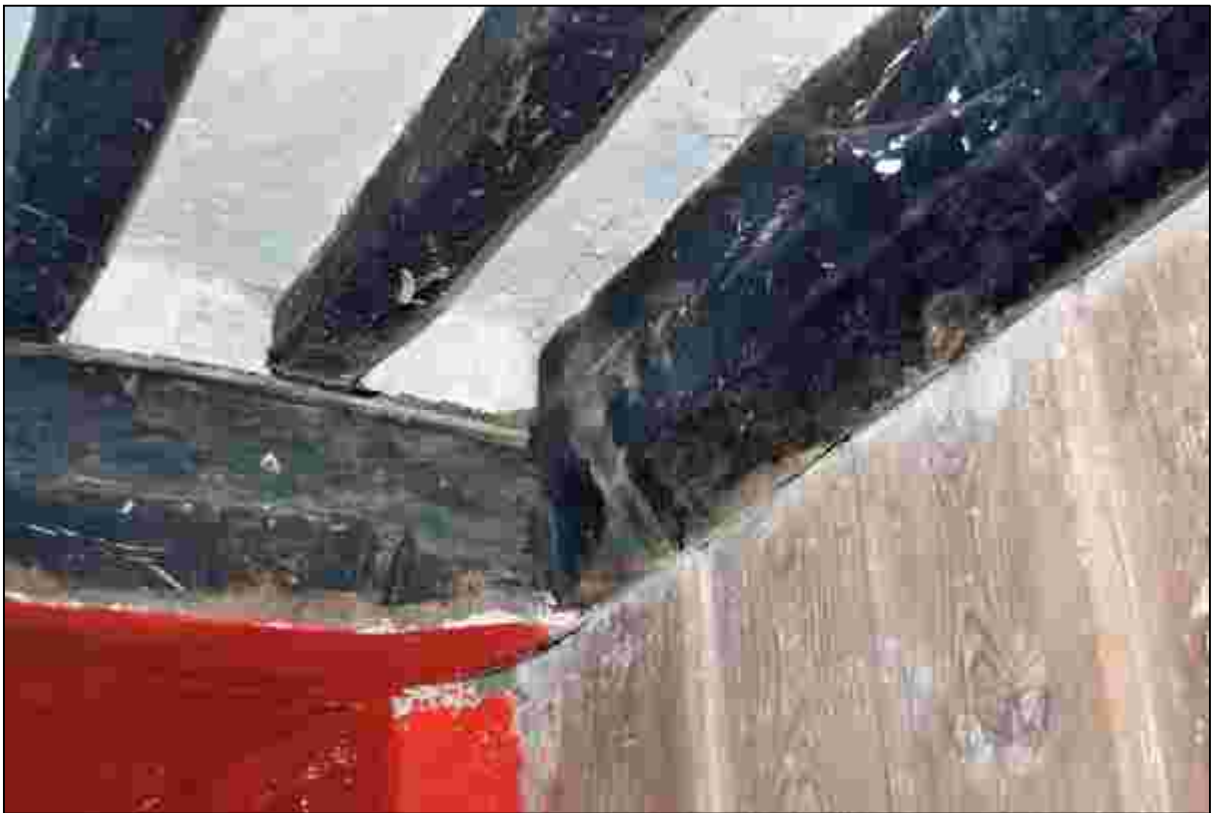
Plate 30: Bar stops on beams in the north eastern corner of the Hall
