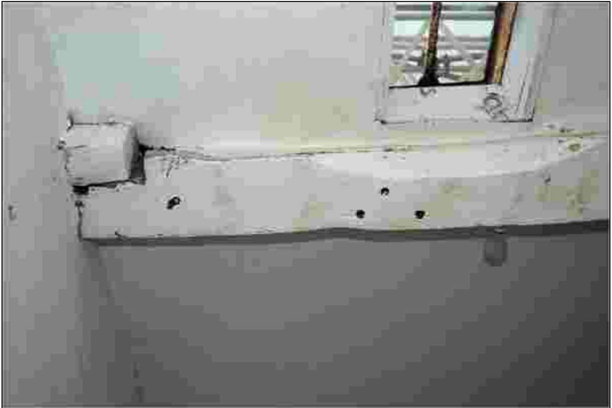
Plate 39: Peg holes for one of the windbraces in the lower, northern purlin
