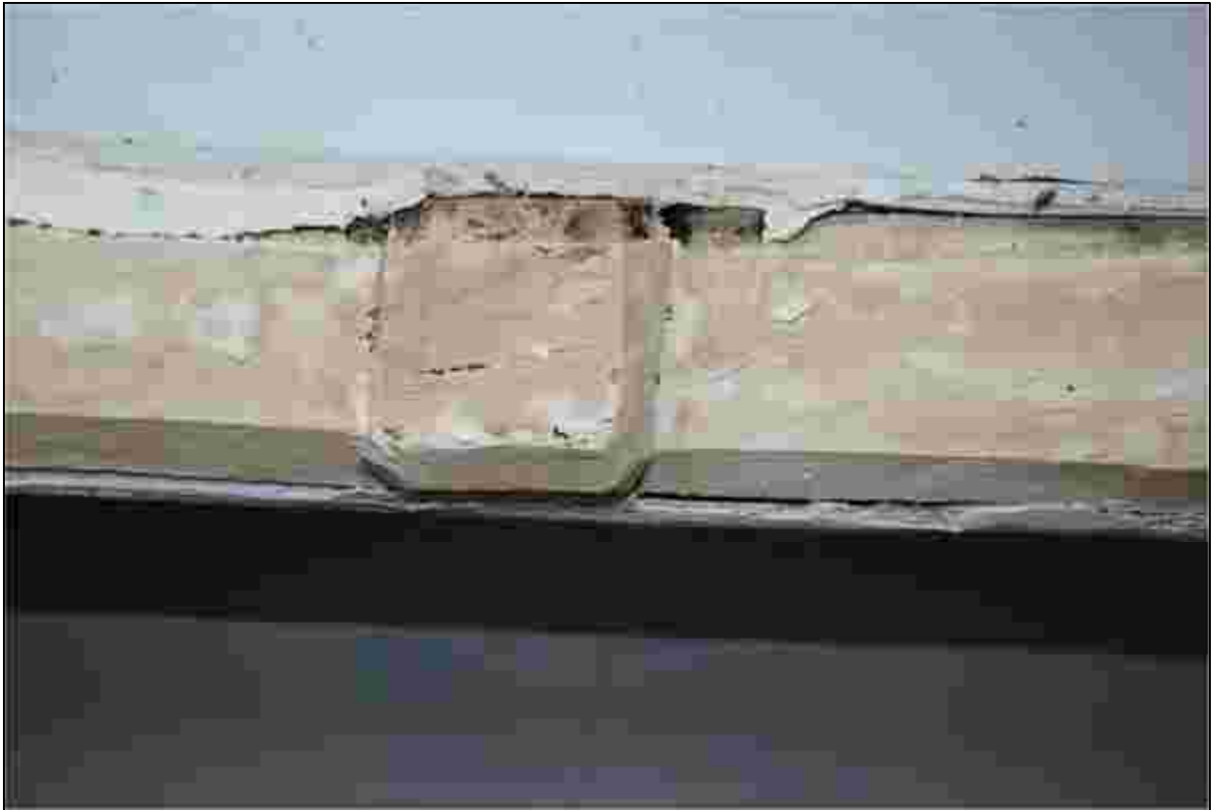
Plate 53: Central boss on Truss 2 from below
