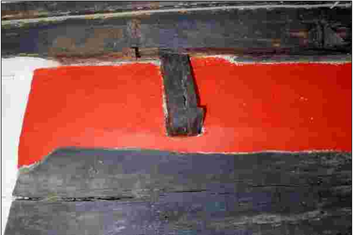
Plate 33: Southern strut above the hearth bressumer
