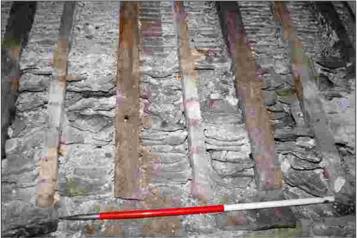
Plate 77: Deposit of moss slates over the northern wall plate
