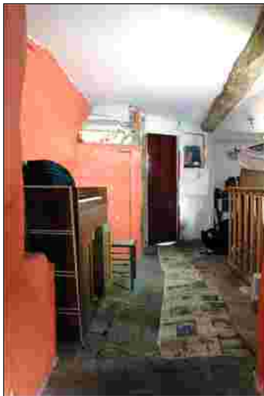
Plate 24: The position of the cross passage showing the protrusion of the back of the chimney breast
