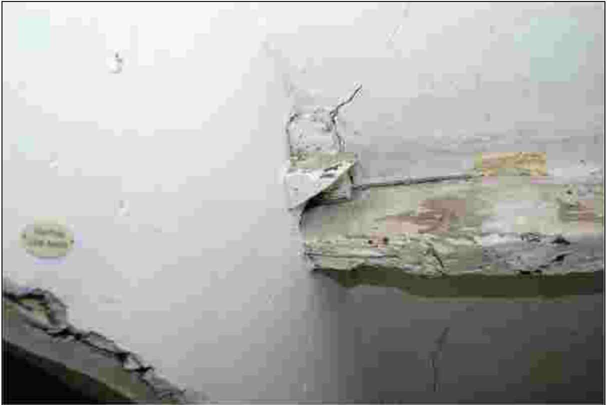
Plate 55: Overlap of the purlin on the northern side of Truss 2
