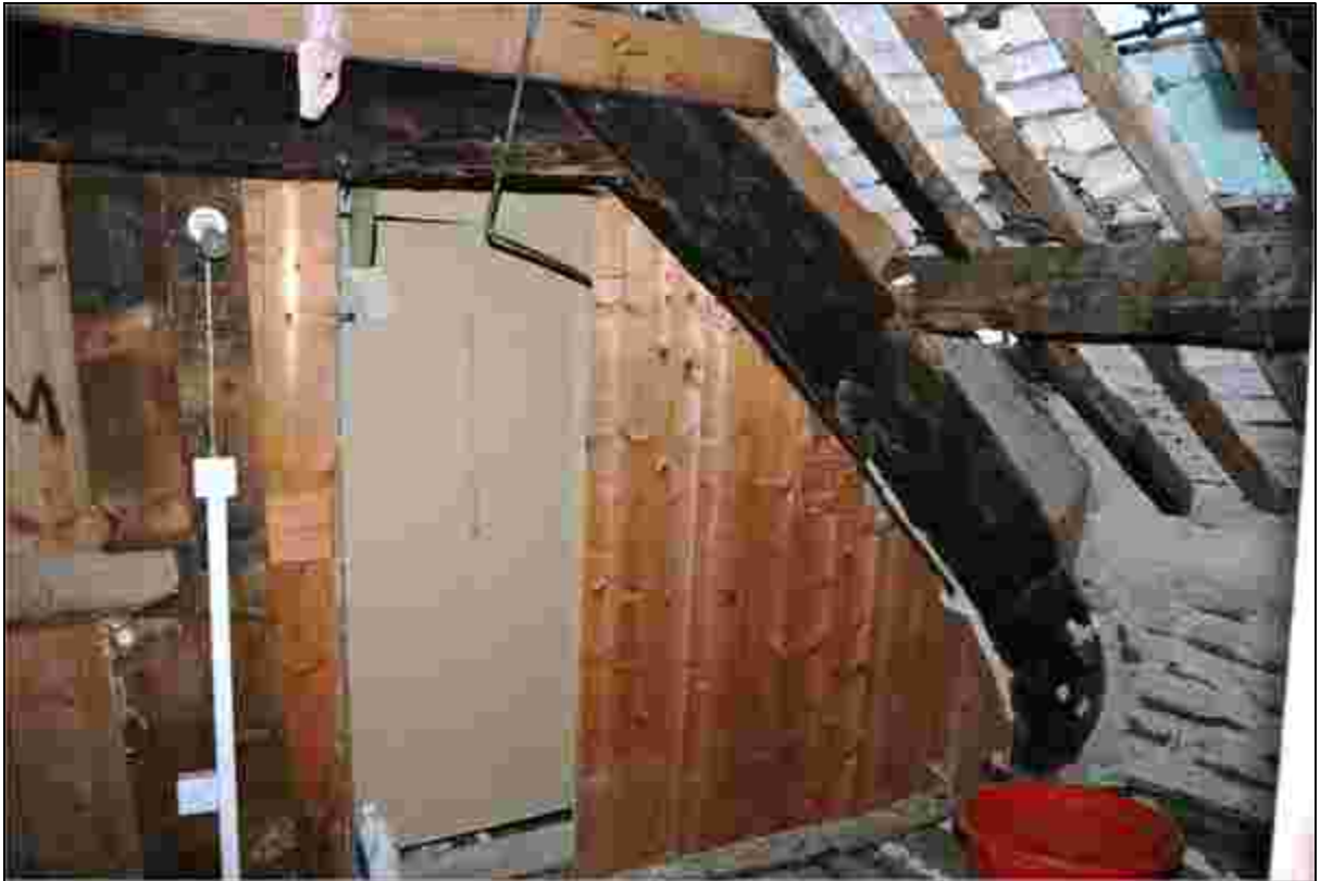
Plate 61: Northern principal rafter of Truss 3
