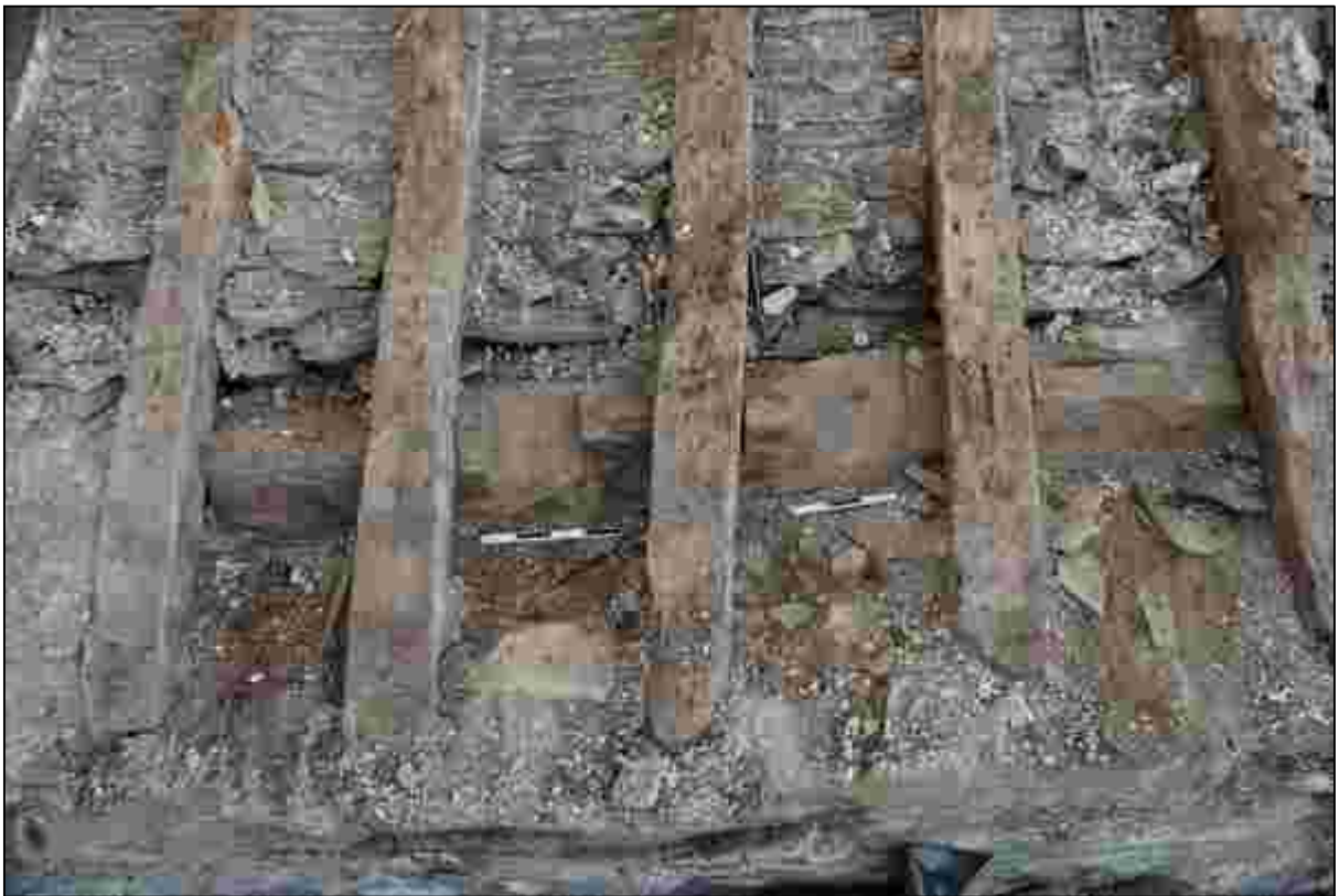
Plate 76: Trenches for earlier common rafters
