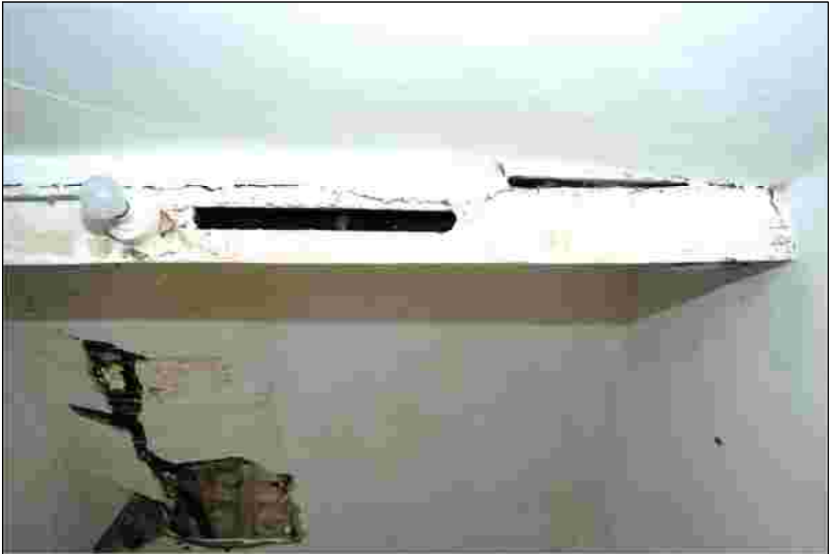
Plate 37: Slot for a windbrace below the lower northern purlin
