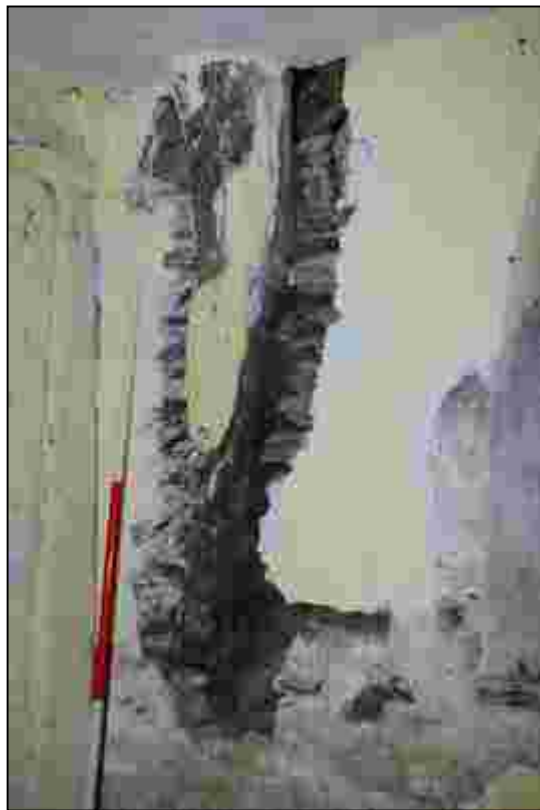
Plate 90: The norther blade of Truss 3 extending into the wall
