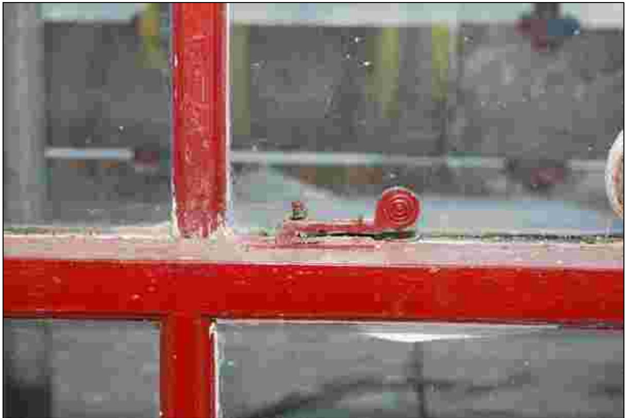
Plate 45: Latch on window in Bedroom 1
