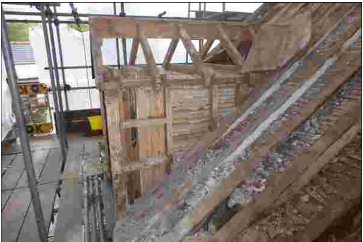
Plate 82: Structure of the dormers
