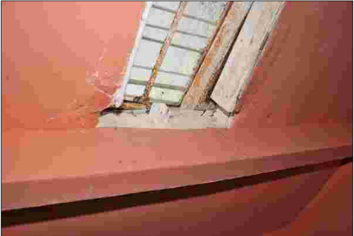
Plate 59: Sawn off common rafter for the ceiling light in the Bathroom
