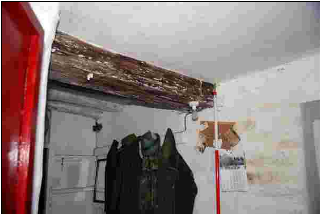
Plate 22: Head rail for the cross passage partition in the lobby
