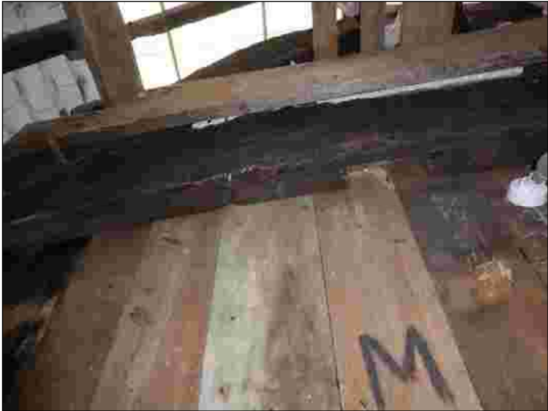
Plate 63: Mortice below the collar of Truss 3
