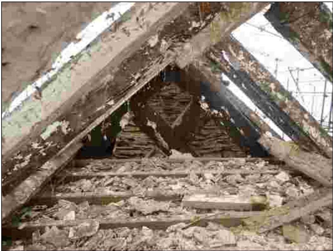
Plate 70: Top of Truss 2
