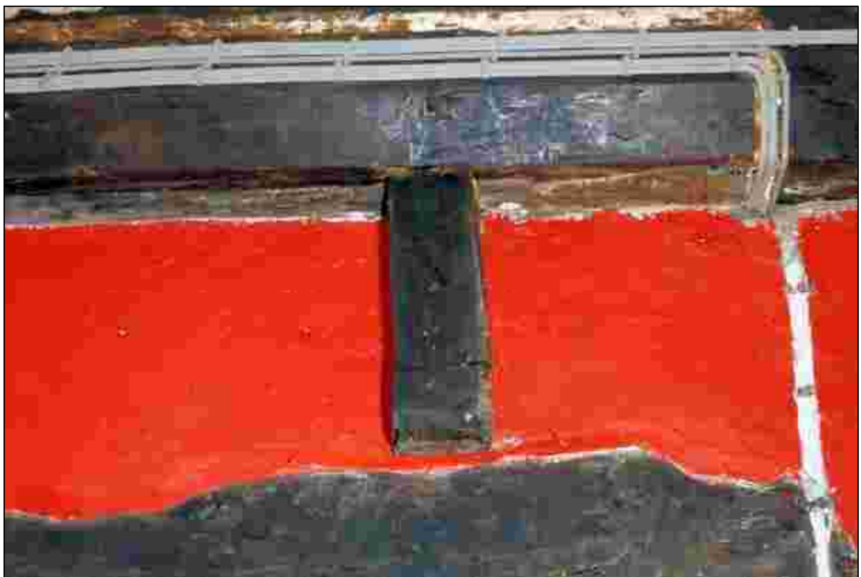
Plate 32: Northern strut above the hearth bressumer
