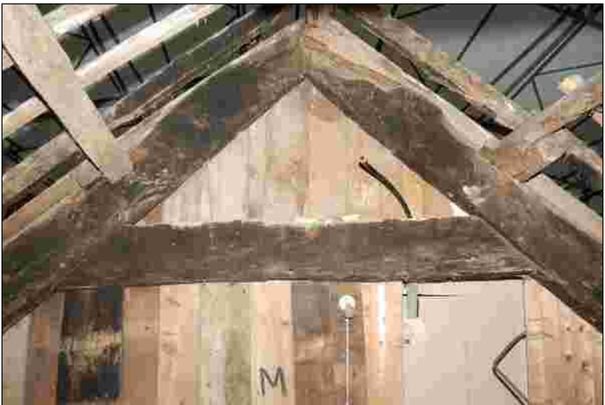
Plate 62: Top of Truss 3
