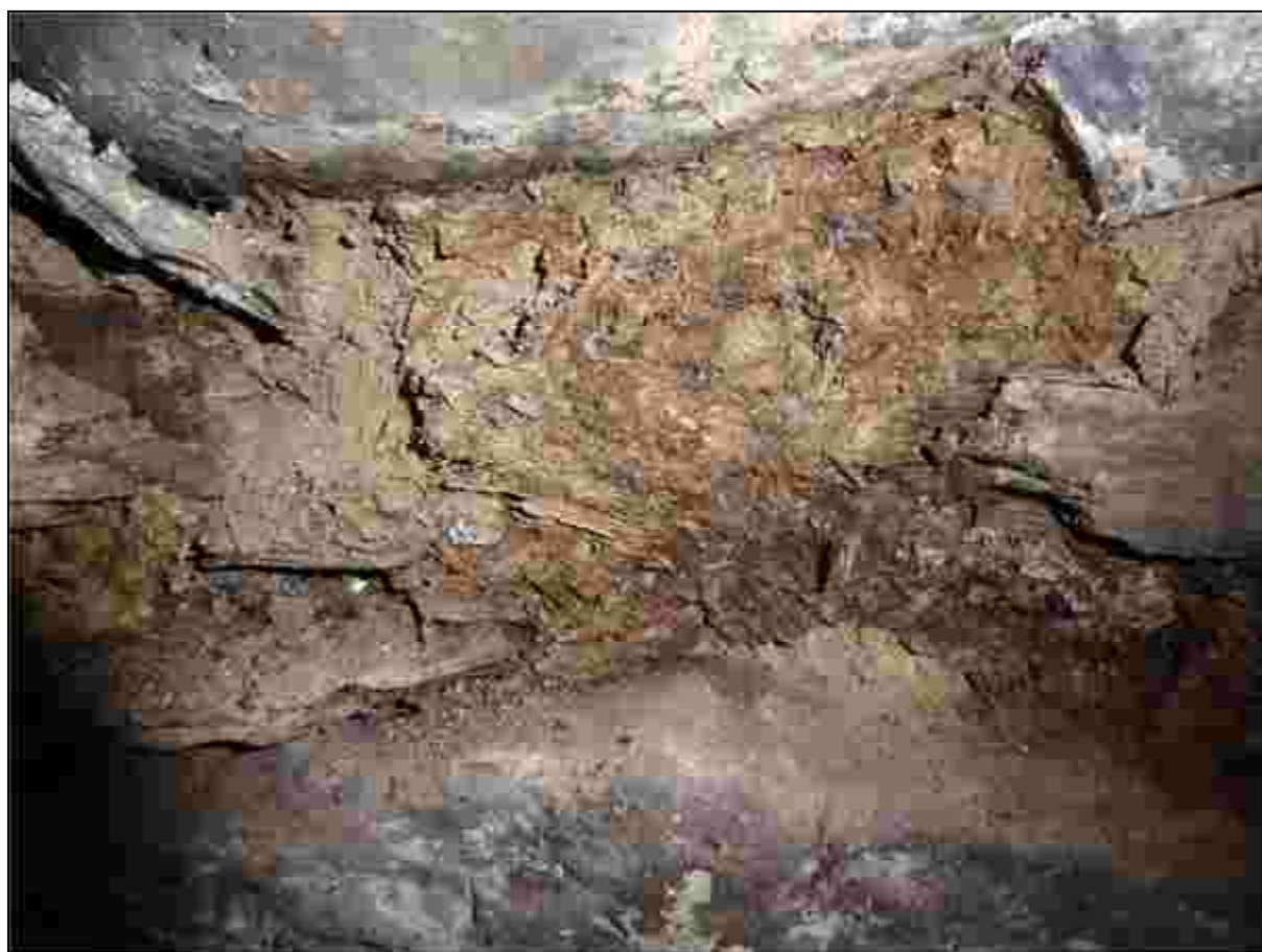
Plate 92: Detail of the earth bonding in the wall near the southern blade of Truss 3
