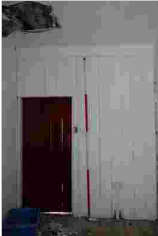
Plate 41: Partition dividing the landing from Bedroom 2
