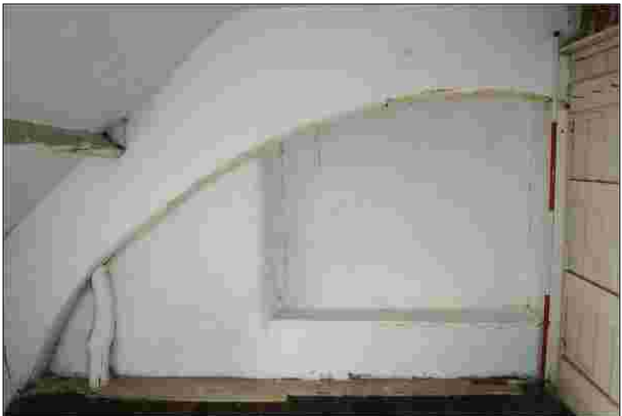
Plate 50: Truss 2 in Bedroom 4
