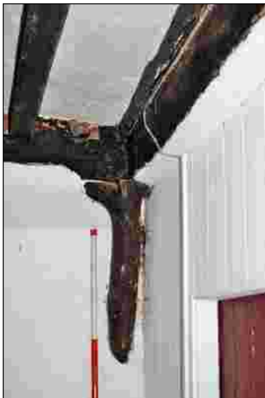
Plate 34: Inserted strut in the south western corner of the hall
