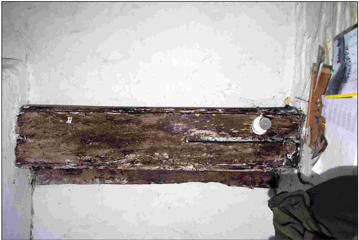
Plate 23: Detail of the slots for the partition.
