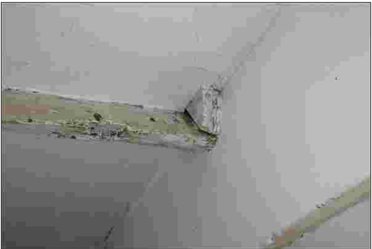
Plate 54: Overlap of the purlin on the southern side of Truss 2
