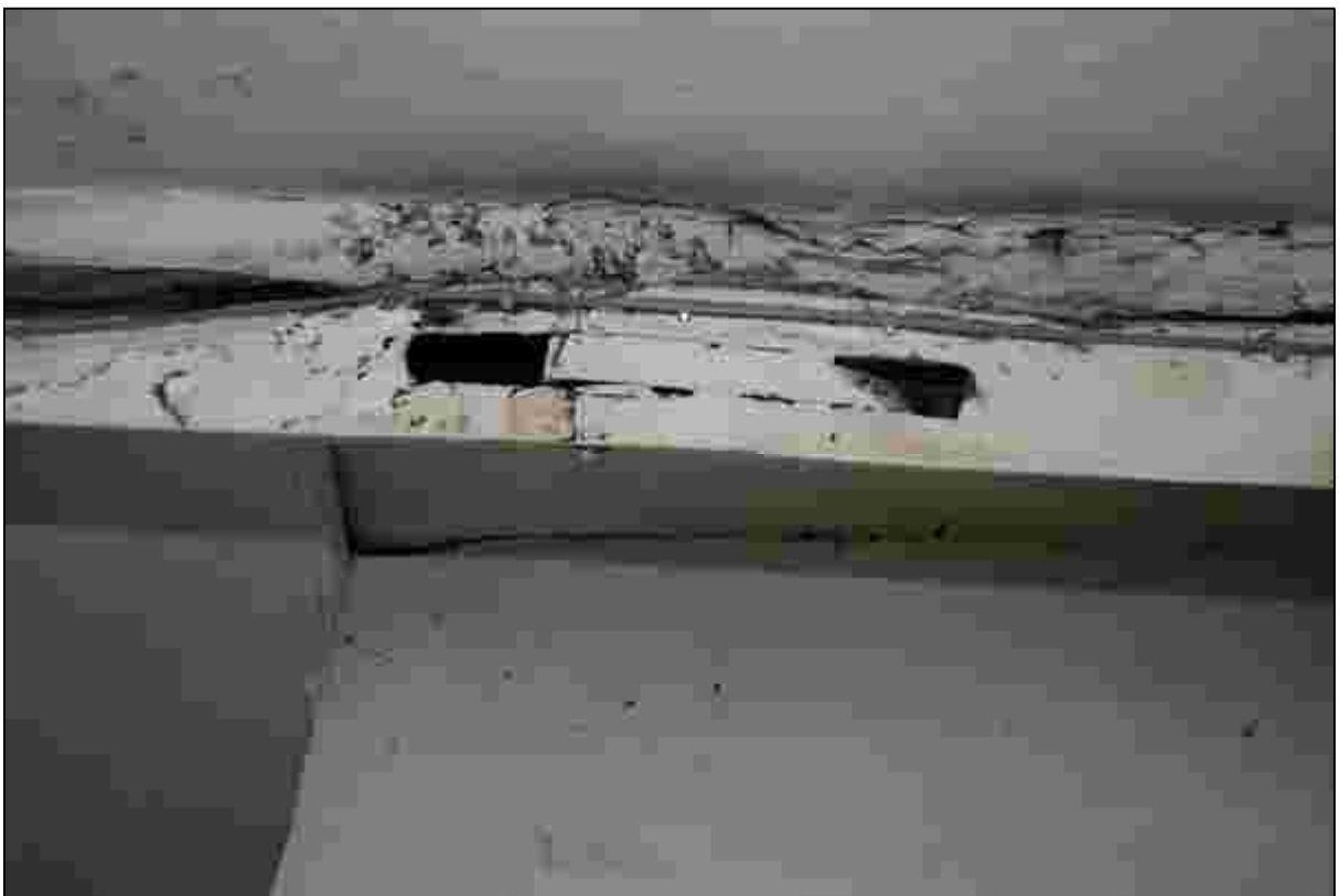
Plate 38: Slot for a windbrace below the lower northern purlin
