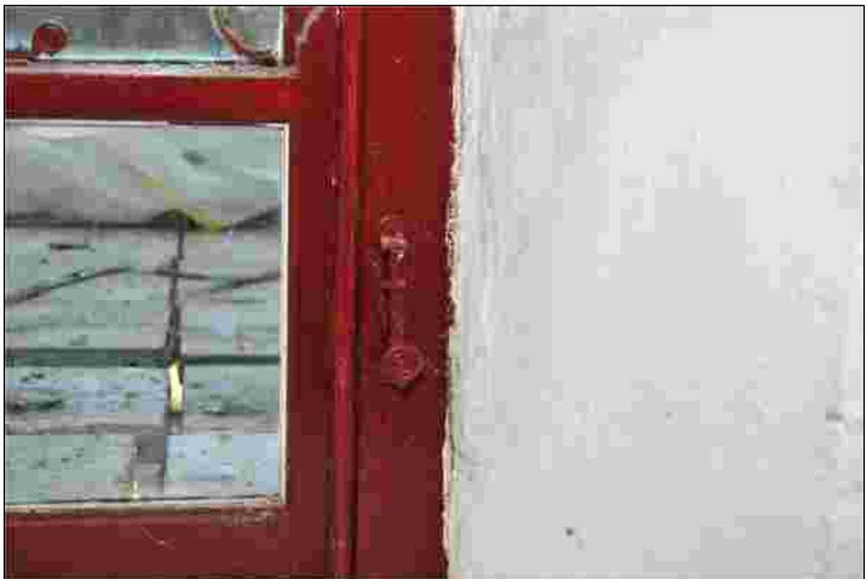
Plate 44: Fitting on the window in Bedroom 1
