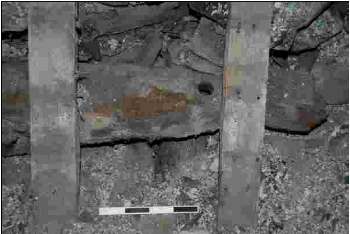
Plate 73: Peg hole at the eastern end of the southern wall plate
