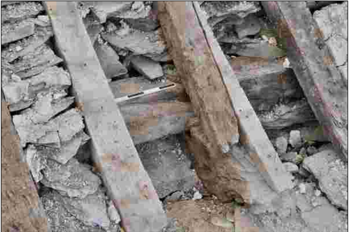
Plate 75: Lap joint between the timbers forming the northern wall plate
