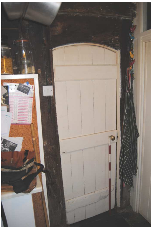
Plate 22: Door to [GF03] with raised head.
