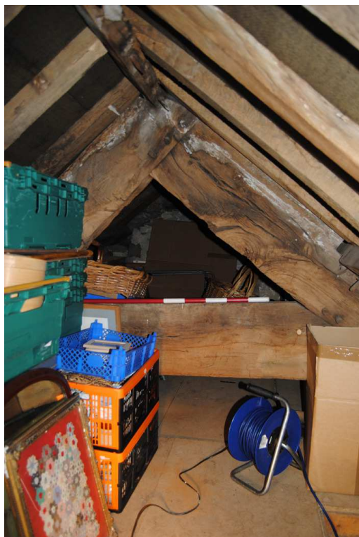
Plate 33: Apex of truss T1 looking south.
