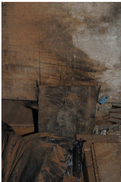
Plate 37: Truss T2, halved and lapped stud.
