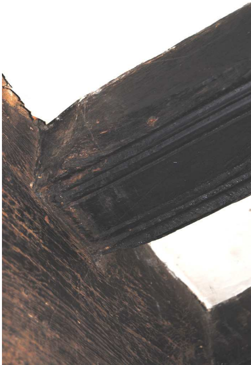
Plate 18: Detail of moulded common joist, [GF02].
