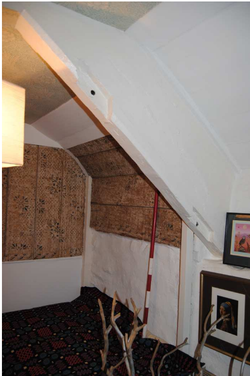
Plate 31: [1F04], west principal of T2 displaying lap joints for former vertical studs.
