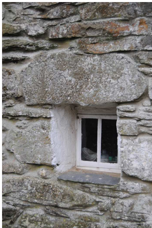
Plate 4: Primary window with monolithic head.
