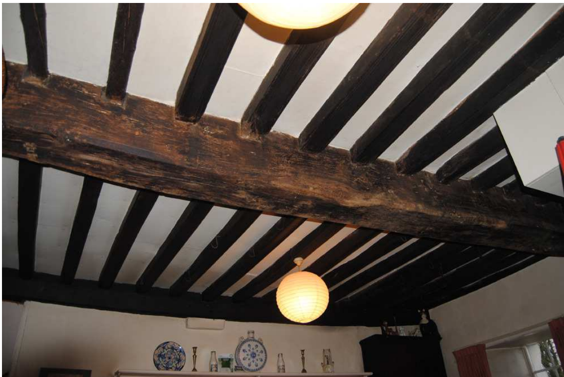
Plate 17: Ceiling structure over [GF02].
