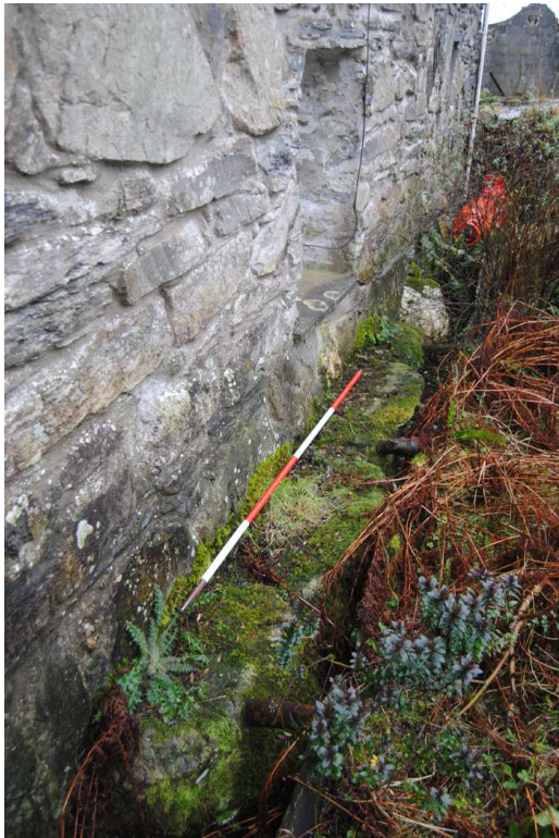
Plate 6: Offset boulder footing to west elevation.
