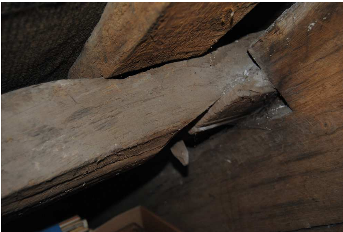
Plate 38: Detail of splayed scarf at T2 (W).
