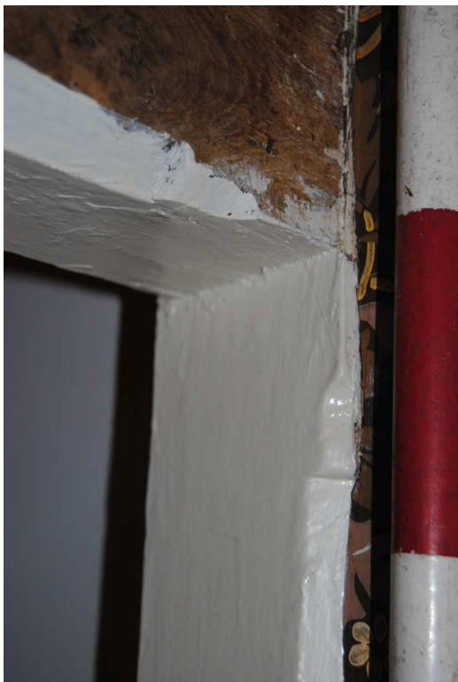
Plate 26: Ogee-stopped door jamb and head below T2.
