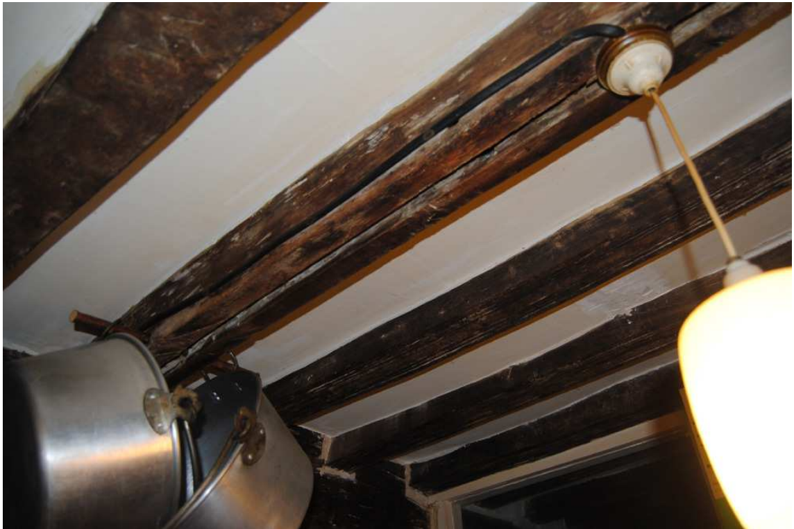
Plate 21: Ceiling structure of [GF03] with redundant mortices and groove indicating former lateral partition; NB: common joists to east are moulded, those to west are plain.
