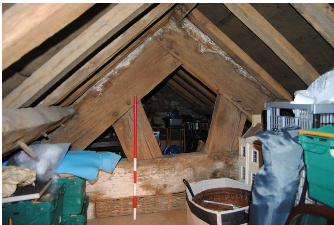
Plate 35: Apex of truss T2 looking north.
