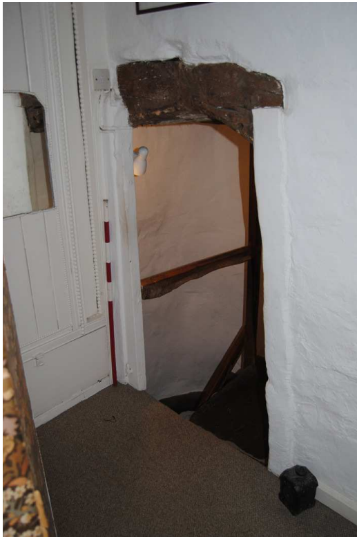
Plate 24: Head of winder stair.
