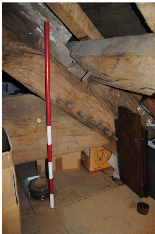
Plate 34: Truss T1, multi-pegged collar joint.
