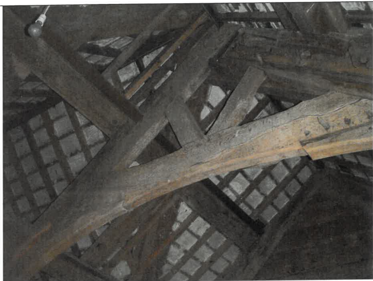
Plate 5 Truss T1, from west
