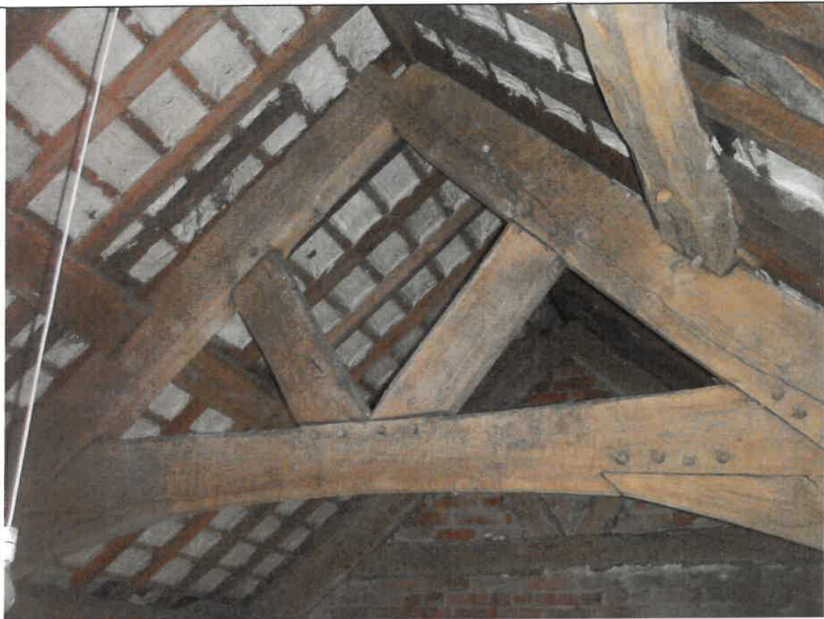
Plate 11 Truss T7, looking north (in north-west wing)
