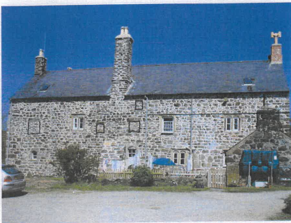
South elevation, marked up to show more clearly the blocked windows and the horizontal line at window head level at the east end
