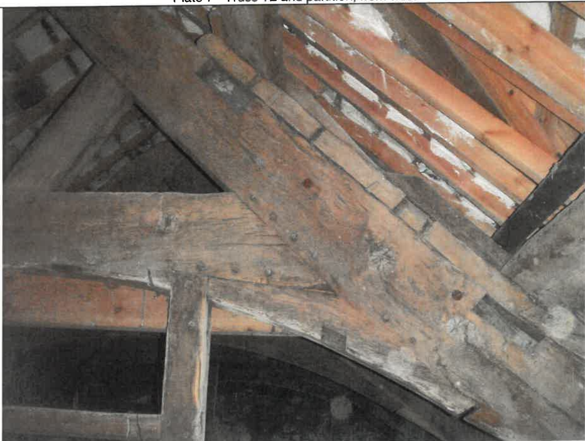
Plate 8 Truss T4, from east
