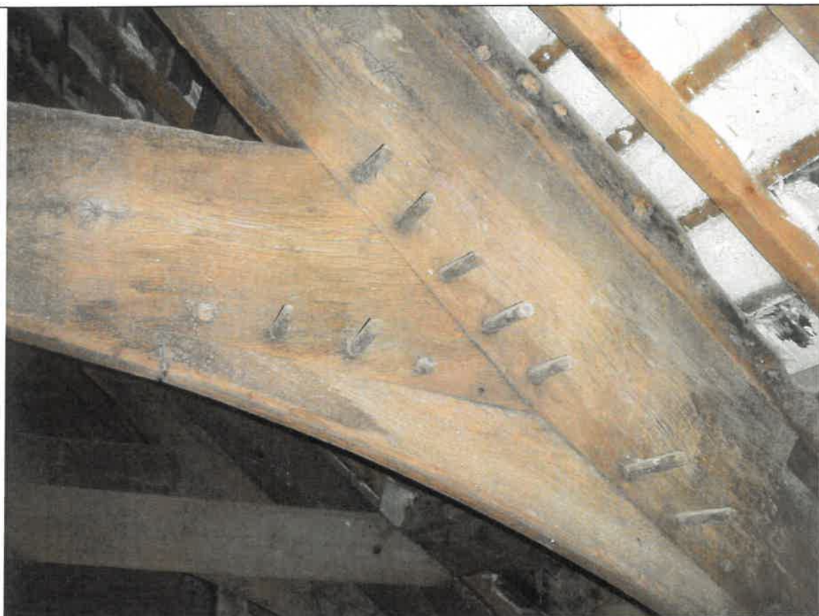
Plate 9 Truss T3, from west, showing pegged joint
