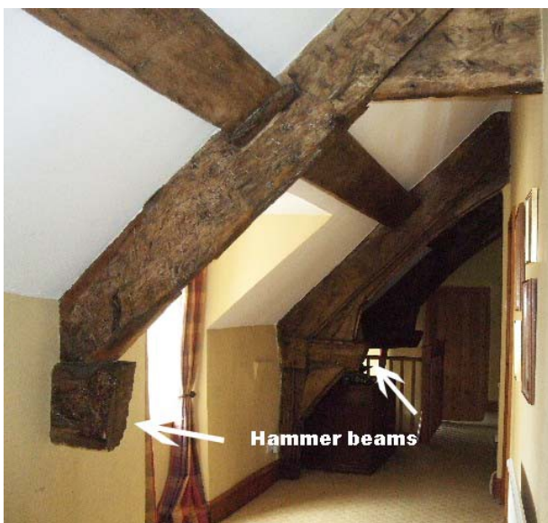
The hammer beams
