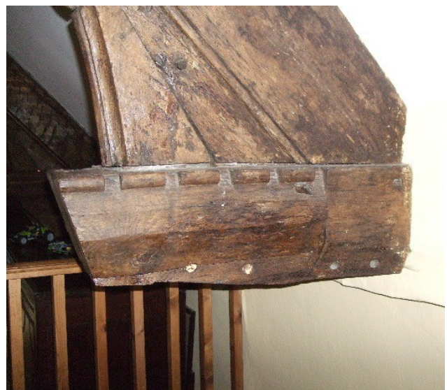
The hammer beams
