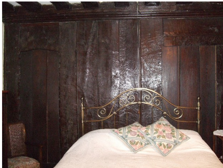
Post and panel partition in the solar
