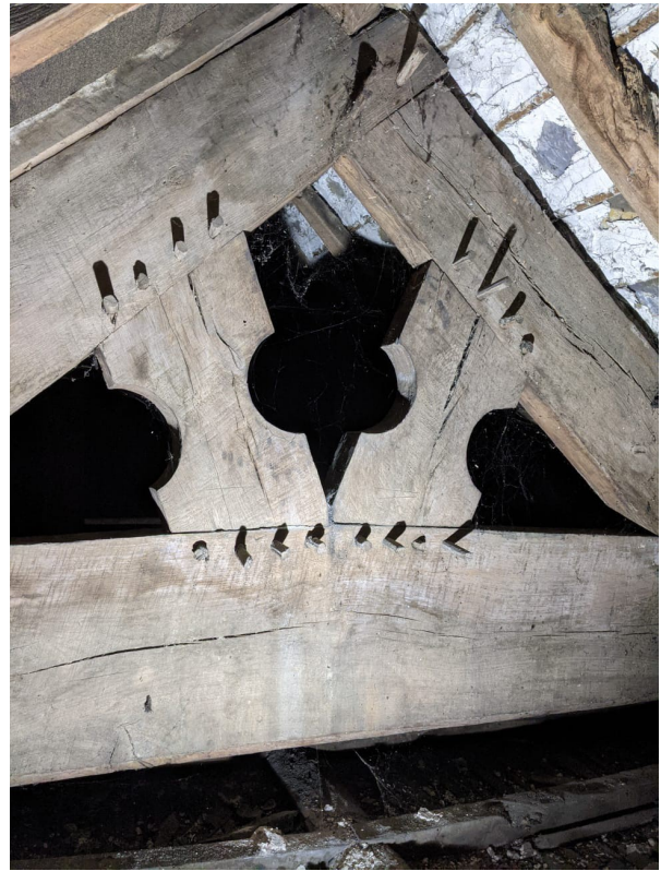
Roof timbers, showing cusing and pegging.
