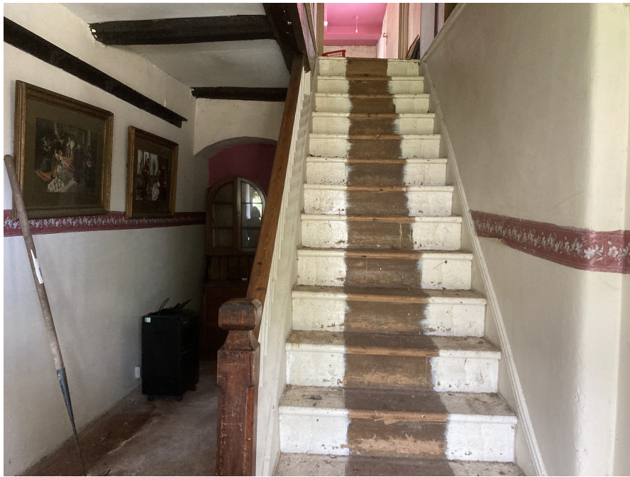
The inserted stairway and later wall to the left.
