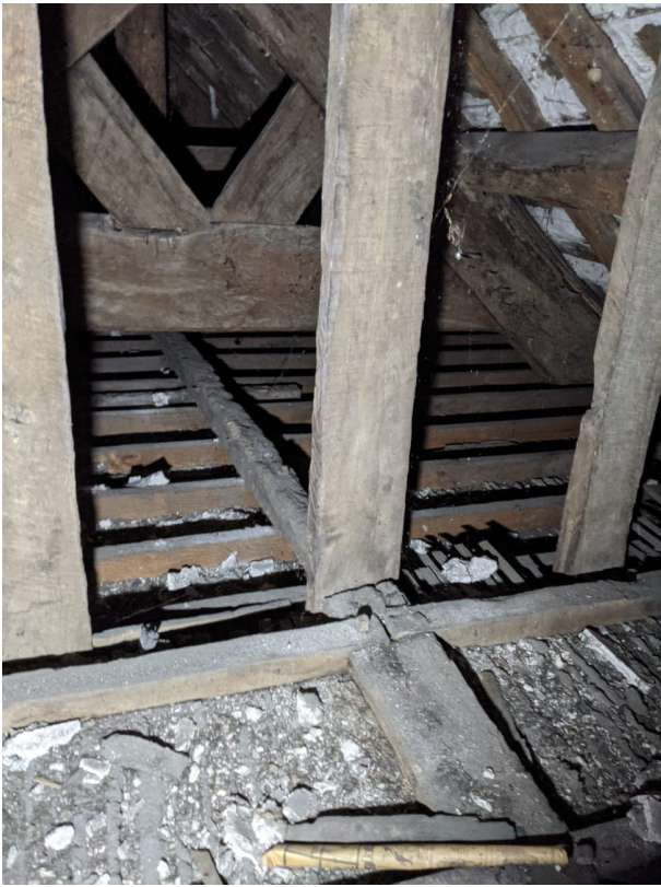
Roof timbers, showing cusing and pegging.
