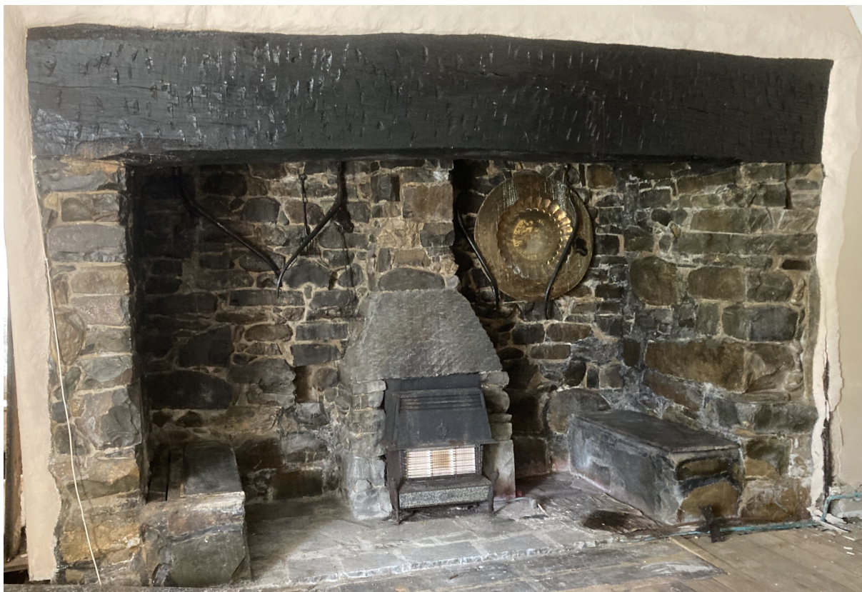
The large inglenook fireplace with stopped-chamfered inglebeam.
