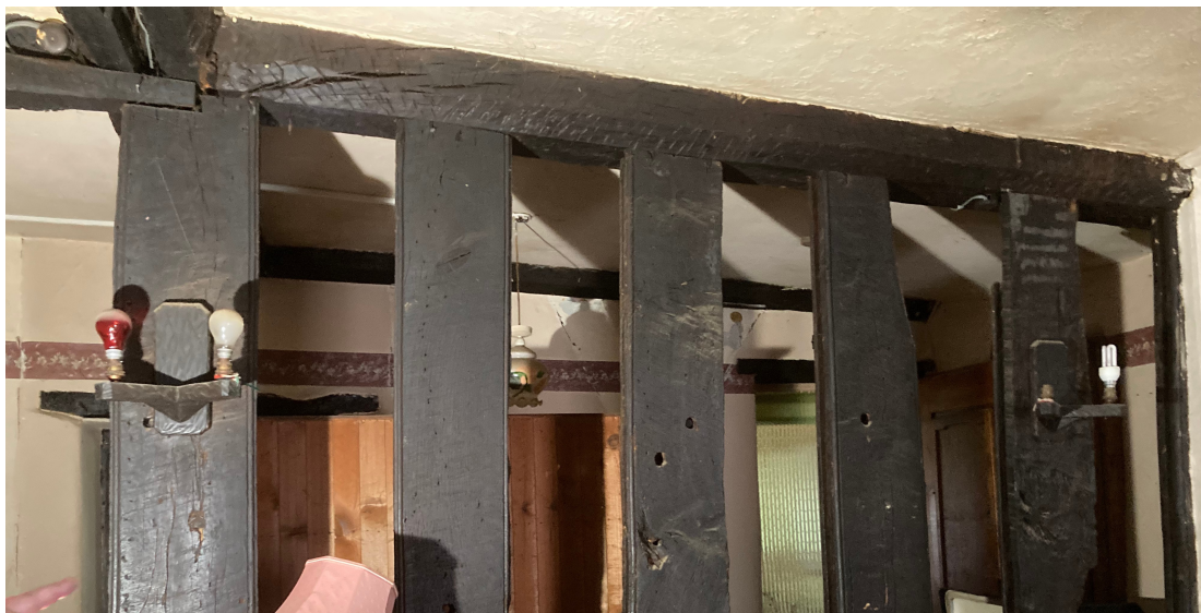
The surviving uprights of a post and panel partition between the service rooms.
