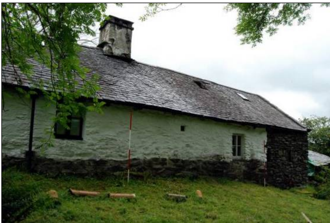
Plate 4: Rear elevation looking NE
