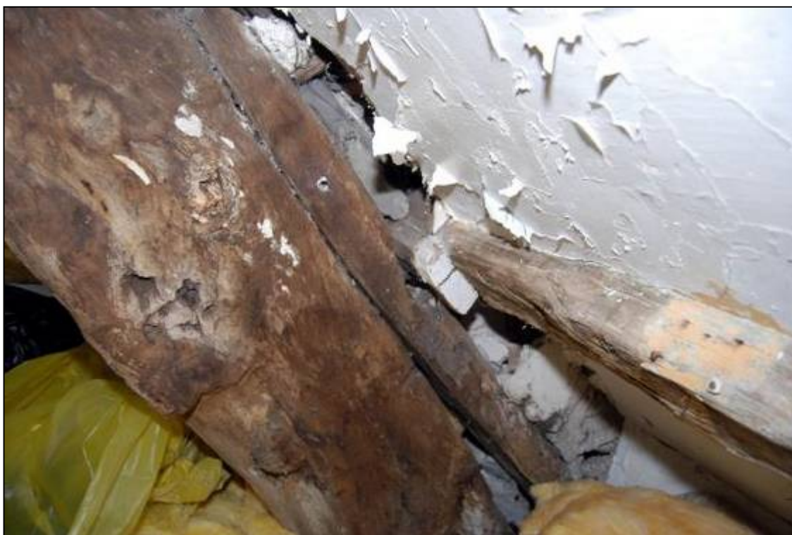
Plate 38: The secondary rafter, northern side of Truss 2
