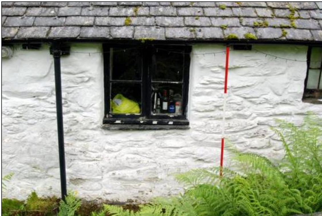
Plate 8: Partially blocked doorway in the front elevation
