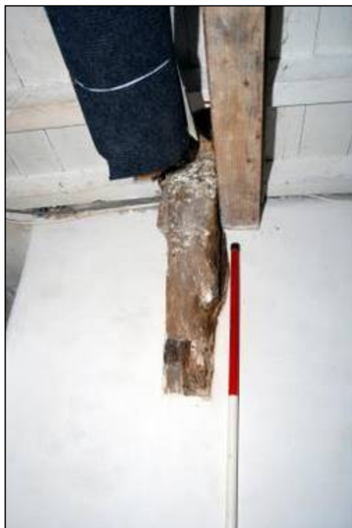
Plate 28: The northern cruck blade in the lower western room
