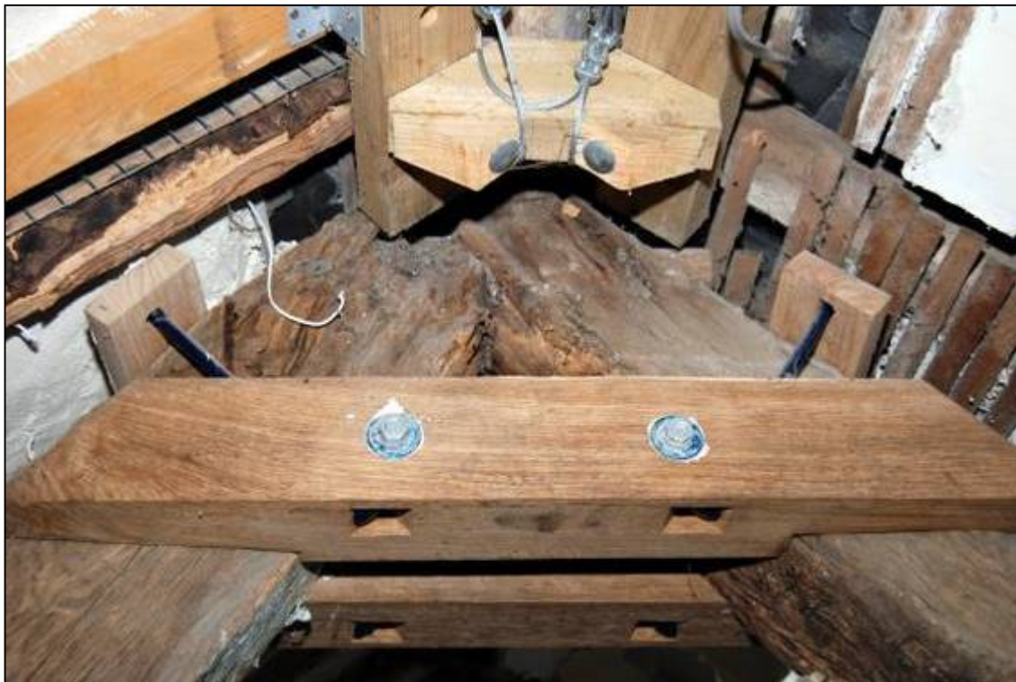
Plate 12: Peak of Truss 1
