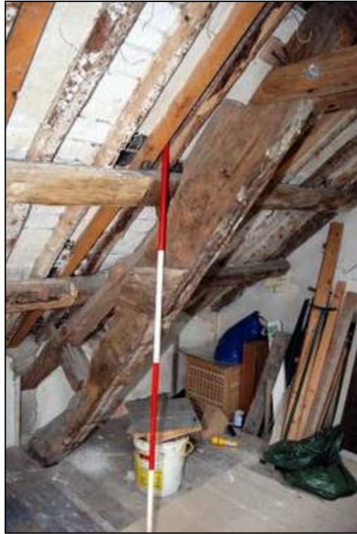
Plate 15: The southern principal rafter of Truss 1
