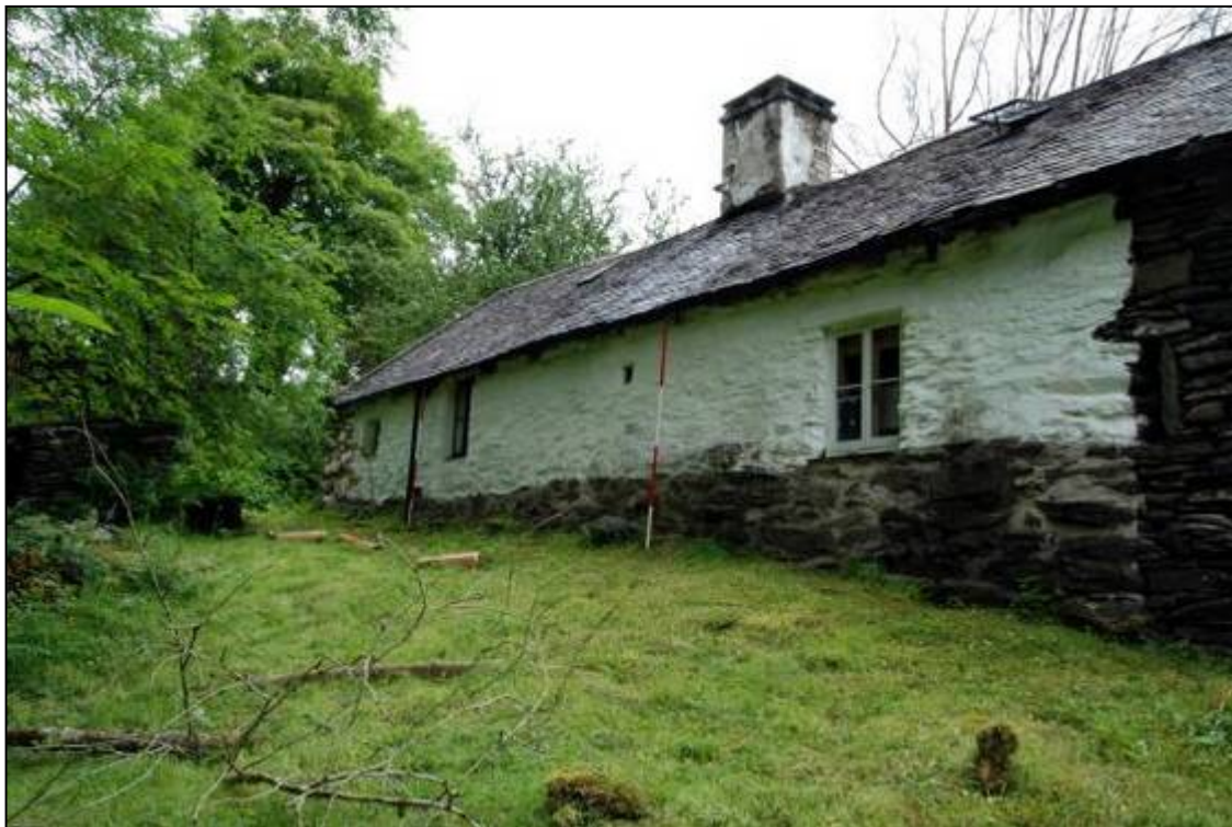
Plate 3: Rear elevation, looking NW
