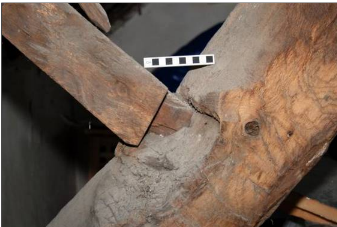
Plate 22: Detail of the joint between the southern principal rafter and the support for the secondary rafter of Truss 1
