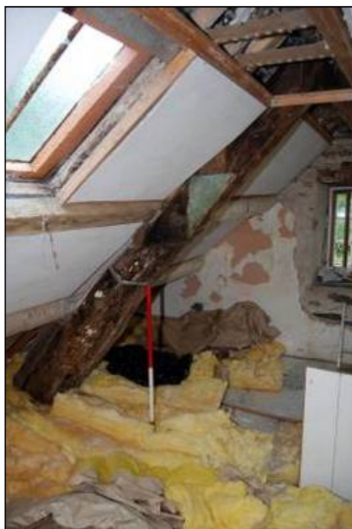
Plate 34: The southern blade of Truss 2
