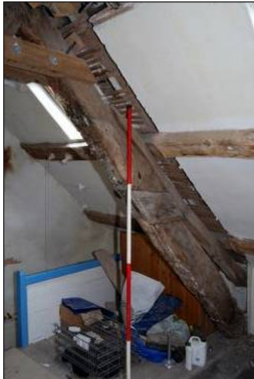
Plate 13: The northern principal rafter of Truss 1
