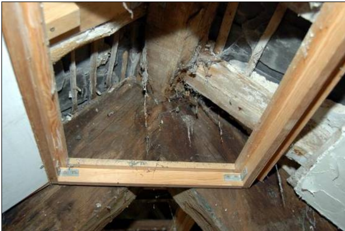
Plate 33: Peak of Truss 2
