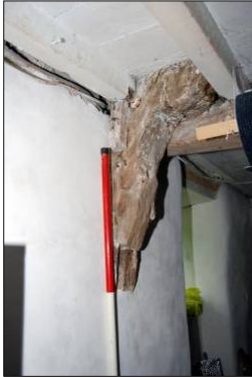
Plate 29: The northern cruck blade in the lower western room, looking NE
