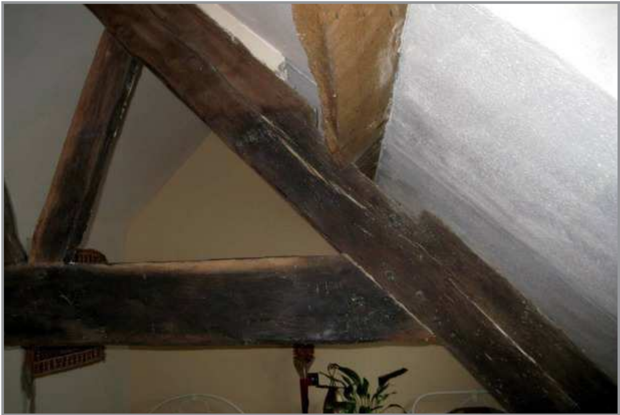
Plate 21: Truss 1 in second floor bedroom. Facing west
