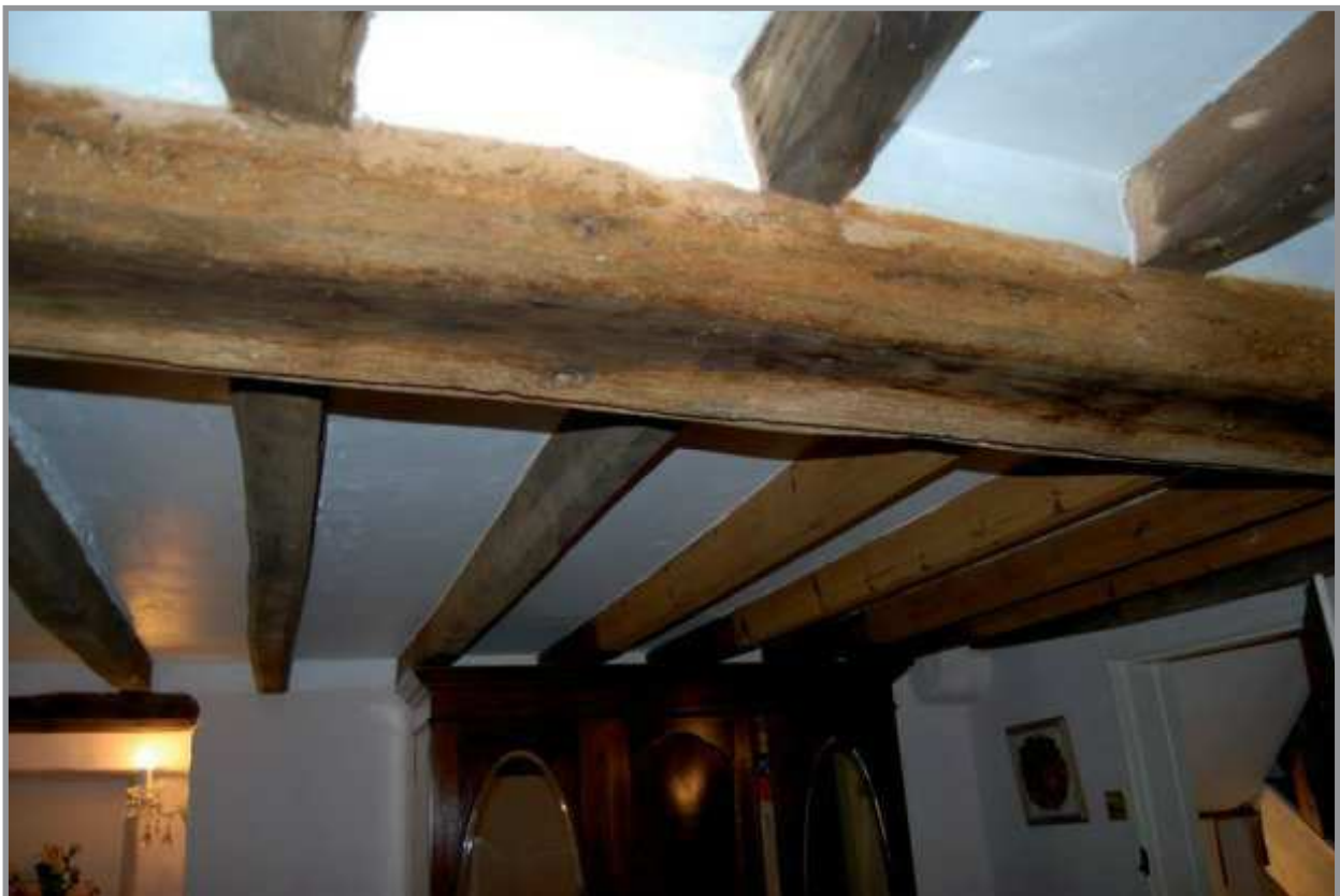
Plate 16: Front bedroom, showing chamfered beam. Facing south
