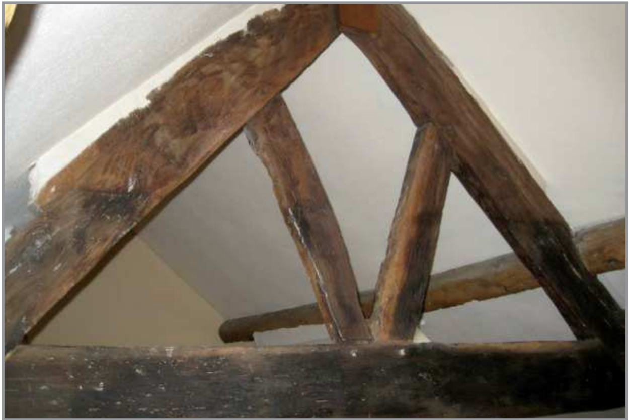
Plate 19: Truss in the cond floor bnt o om. Fach g eat
