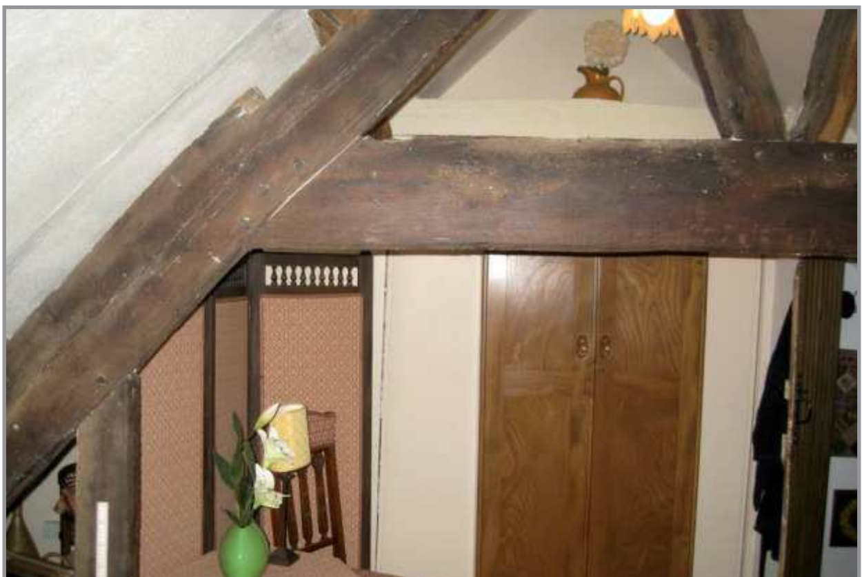
Plate 20: Truss in the cond floor bnt o om. Fach g eat
