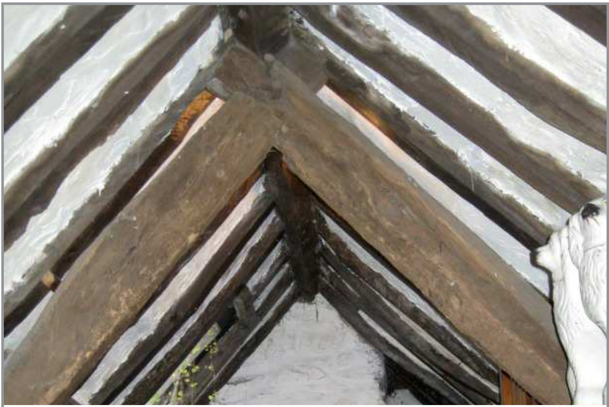
Plate 22: Truss 2 in attic room. Facing south-west
