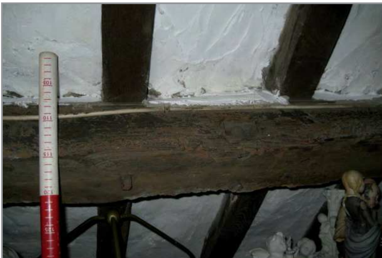
Plate 24: Attic room, showing timber detail. Facing north-west
